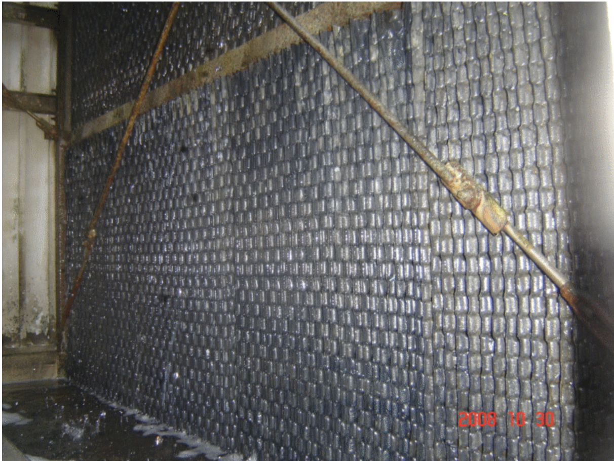
10/30 before use MB ball, there was huge scale everywhere in the radiator.
