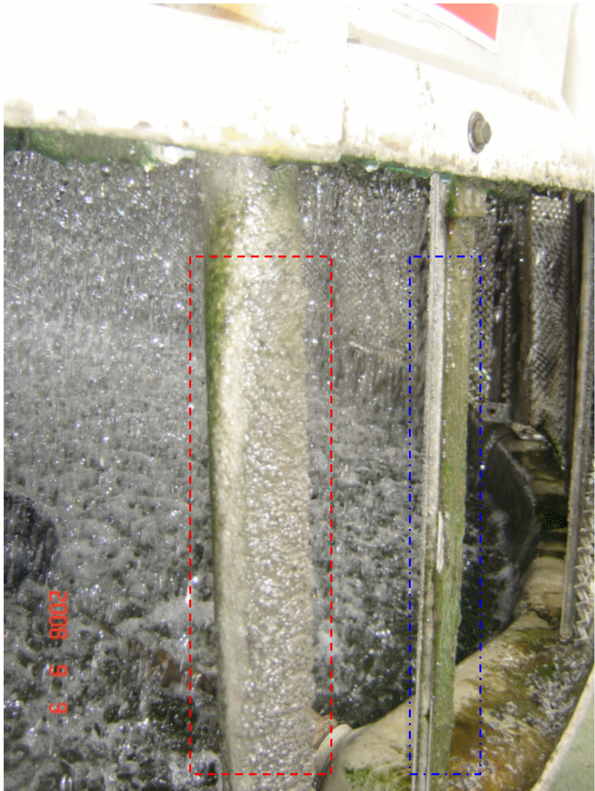
9/9 before use the MB ball, hard scale adhered to the prop stand, it was removed very difficult.
