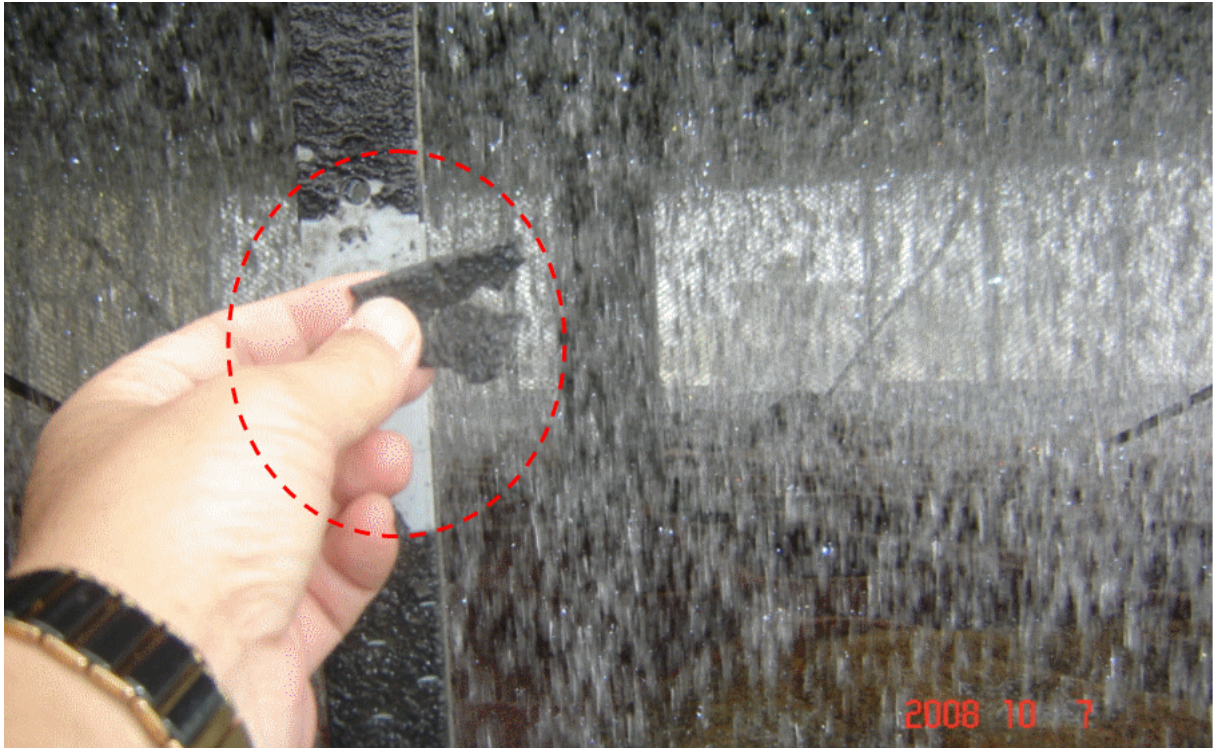
10/7: six weeks later, soften the scale of the prop and removed so easy.
