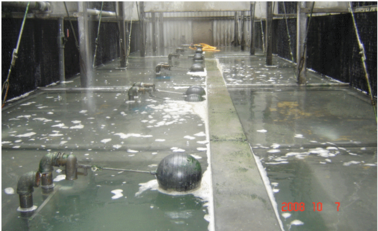
10/7: 5 weeks later, water keep clear, large scales drop into the bottom.
